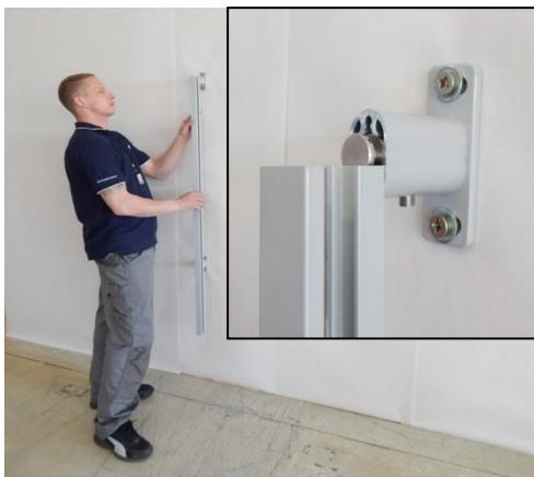
7. Slide the guide rails with rear profile onto the bolts.
