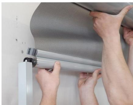
3. Insert bottom bar, antiwind bars and cassette in the guide rail.
