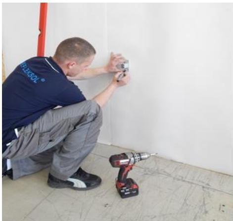
1. Designate spots in the axis of installation of brackets to the base. Put the bracket on the base and mark places for installation holes.
