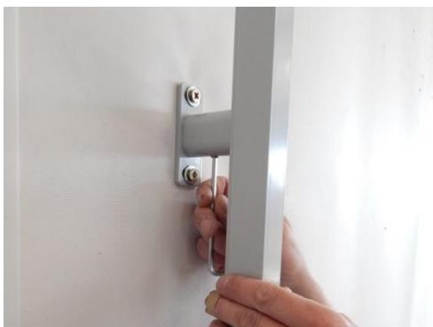
8. Set guide rail in the appropriate position and secure clamping screw in the brackets.
