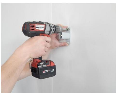
2. Drill holes, then mount the bracket using appropriate fixing system.
